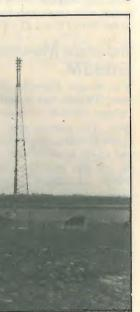
Hedlevhope, the BBC's 500th u.h.f. station, with modular, 3-legged tower, log-periodic aerials and prefabricated building, all of BBC design.
